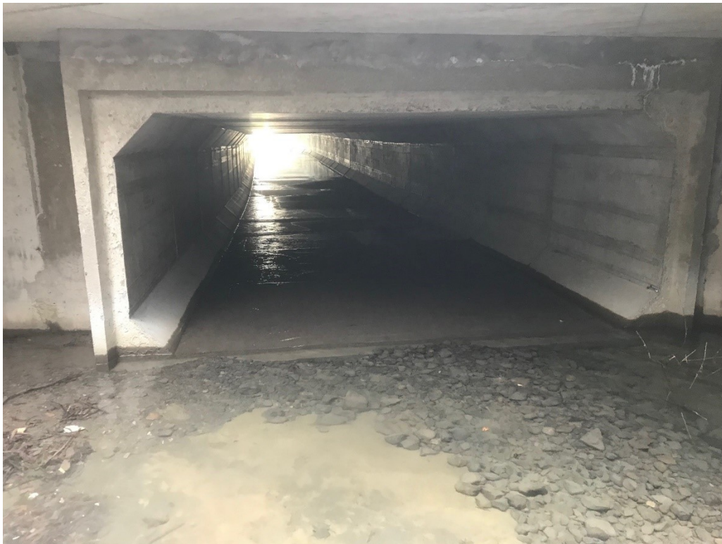
View towards outlet of cleanout chamber (note lip for holding bedload)
