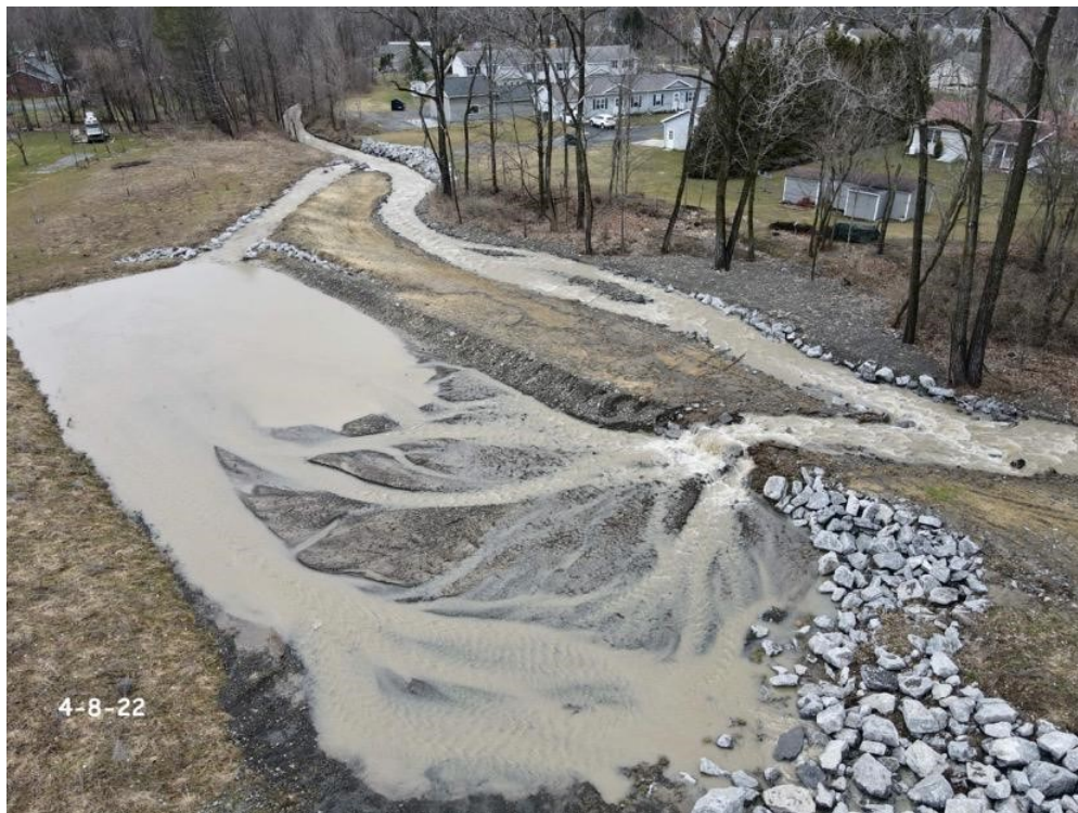
Sediment Basin at work spring thaw 2022
