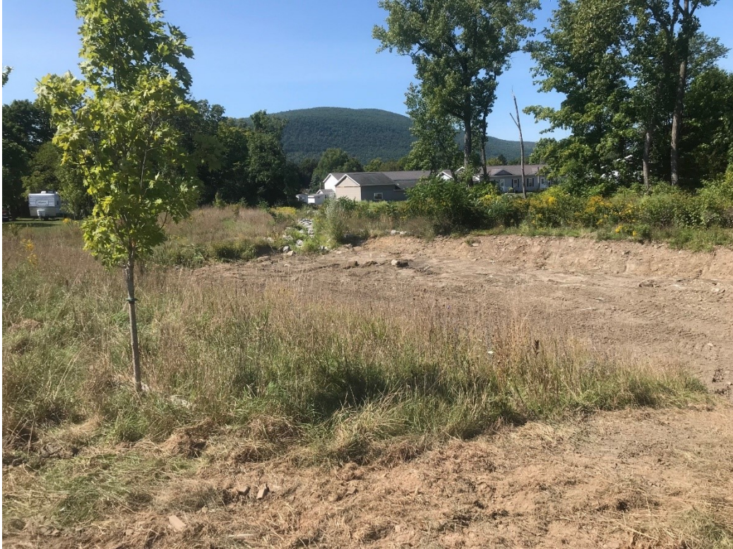
Cleaned out sediment basin 9/5/2024
